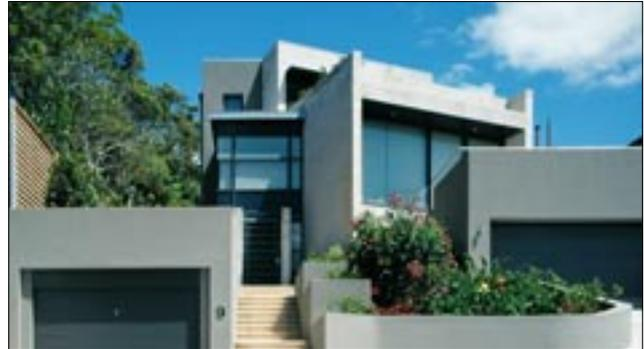
**Rendered brick walls** were chosen for the garage and service spine as a serviceable counter-material to the sandstone.
