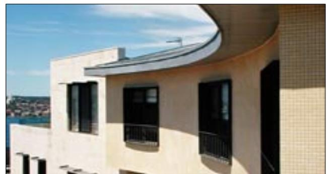
**Extended steel lintels** over the north-facing windows in the sandstone walls also provide solar control, but will admit some summer sun. To avoid all summer heat gain, the lintels would need to be deeper and extend further each side of the window opening. [See: [Shading](#)]
