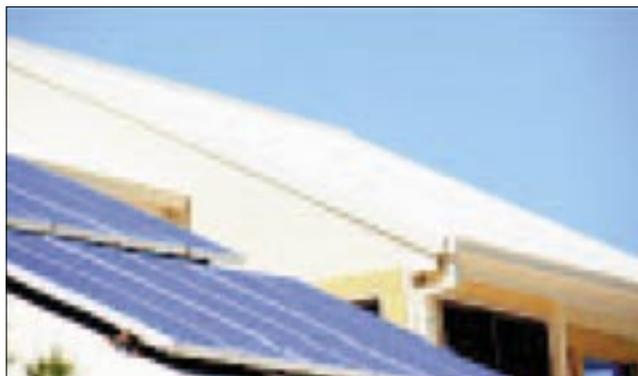
The house is equipped with a 1.6 kilowatt peak grid-connected photovoltaic array installed on the north facing roof, which is pitched at 30° to maximise efficiency of the array in winter.
