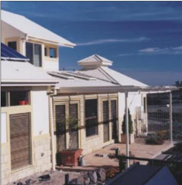
**A solar pergola** ensures the solar court does not overheat and provides a shaded external living area. The reflective solar film on the skylights minimizes overheating of the solar court.
