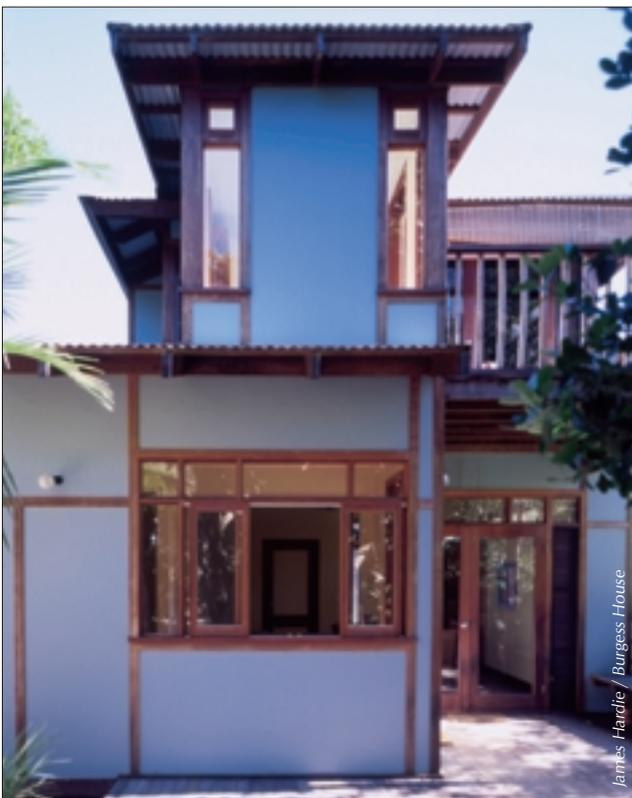
This well insulated home clad in lightweight fibre cement sheeting has low embodied energy and requires little heating or cooling energy to maintain thermal comfort in a warm, temperate climate.
