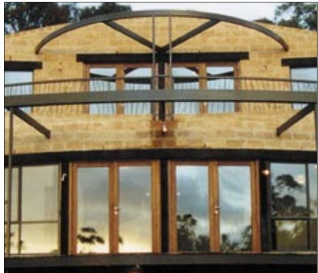
The windows have an external frame of aluminium and a timber frame and reveal internally. These windows provide a low maintenance solution to weathering yet have a significantly higher ‘R’ rating than aluminium-only frames. The windows are all double-glazed and perform as well or better than timber double-glazed equivalents.
