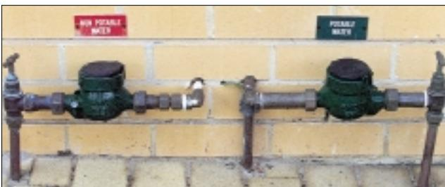
**Rainwater is collected** from all roofs and passes through first-flush pits to storage in four communal in-ground (8 to 10kL) tanks. Pumps and a pressure vessel return this water to supply hot water systems and toilet flushing. Rainwater is therefore used in showering and dishwashing. The rain water tanks are backed up by the mains supply to the site.
