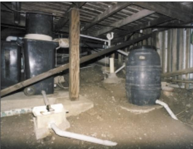
Batch CTs consist of two or more containers that are alternated so that the 'active' container is being used while the pile in the 'fallow' container has time to compost without the addition of fresh excrement and the potential for re-contamination.
