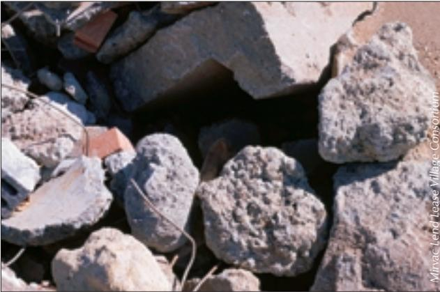
**Break** remnants into small pieces before final set to allow later use as backfill or recycling.
