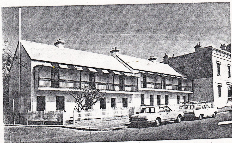
The 'matchbox' terrace at 146-156 St Johns Road, after rehabilitation. This terrace was built in the post-Regency style in the 1840s and is the oldest terrace housing on the Estate.
