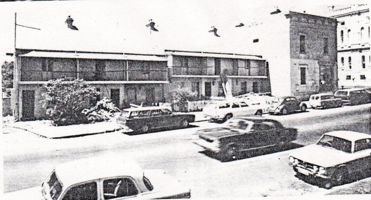
The 'matchbox' terrace at various stages of rehabilitation.
