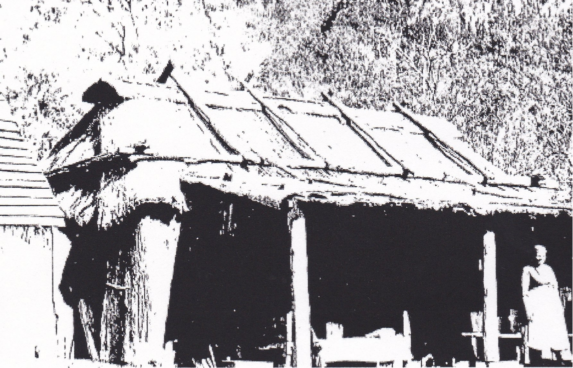
Early settlers house - early 1800s The timber structure on the bark roof is to stop the bark curling up
