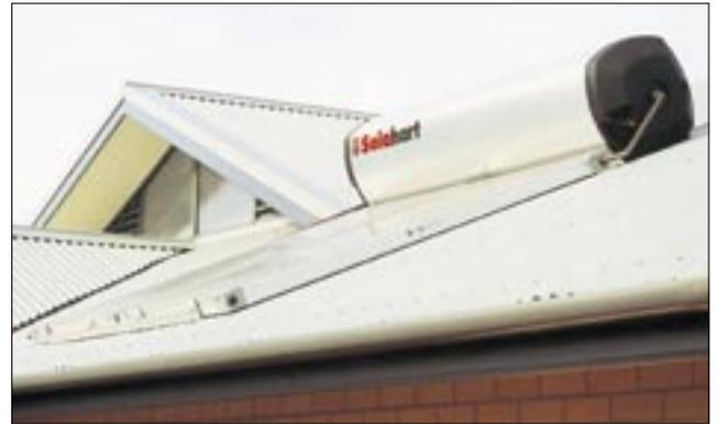
A passive solar thermosiphon hot water system has been mounted on the roof providing free hot water for most of the year. The system operates on the natural recirculating process of thermosiphoning (hot water rising, cold water falling), and therefore does not require a support pump, condenser or compressor. [See: [Solar Hot Water](#)]
