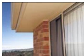
This is not always achievable with standard eave detailing which is flush with the 2100 head. The top 20 percent of this window is in permanent shade.
