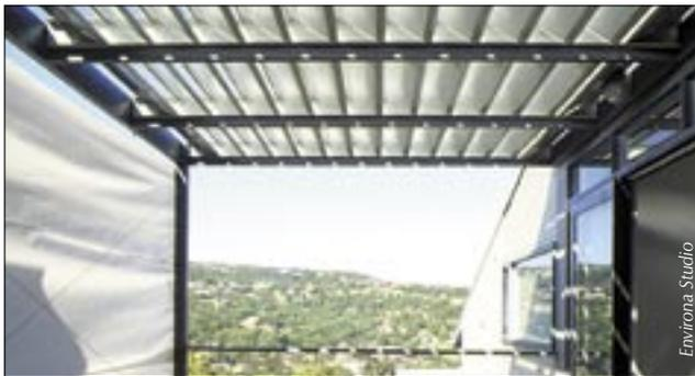
Adjustable shading appropriate for northern elevations includes adjustable awnings or horizontal louvre systems above glazing, and removable shade cloth over pergolas or sails. Shade cloth is a particularly flexible and low cost solution.
