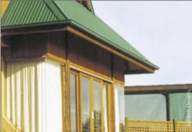
Above, standard 2100 high doors are shaded by a 1000 eave (including gutter) set 300 above the head. Note the sun angle at midday in mid winter is above the glass line. This configuration provides full shading to glass from late October to late February at latitude 35°S (near Canberra) and is appropriate for a higher altitude cool climate winter.
