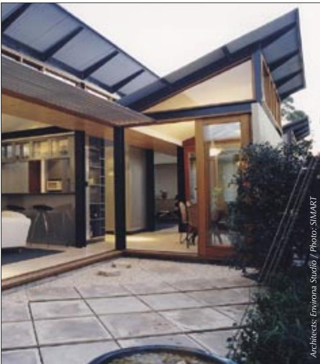
Above, north facing upward raked eaves allow full exposure of glass to winter sun and shade larger areas in summer, without compromising the solar access of neighbours to the south. This inner city terrace in Sydney uses an upward raked eave to passively shade highlight windows. A separate horizontal projection of louvres shades lower glazing. This allows 100 percent winter solar access and excludes all sun between the spring and autumn equinoxes.
