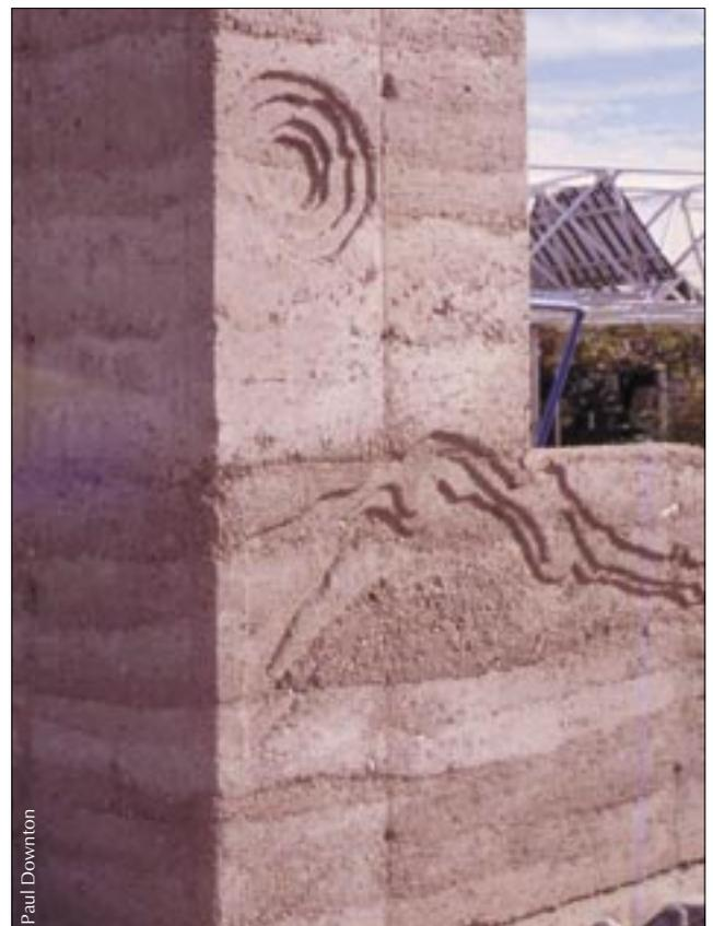
*Unusual finishes can be achieved by including shapes in the formwork that can be released after the wall has been rammed. This sample wall is at the Environmental Research Laboratories in Tucson, Arizona. Other possibilities include embedding rocks and other objects in walls for aesthetic effect.*
