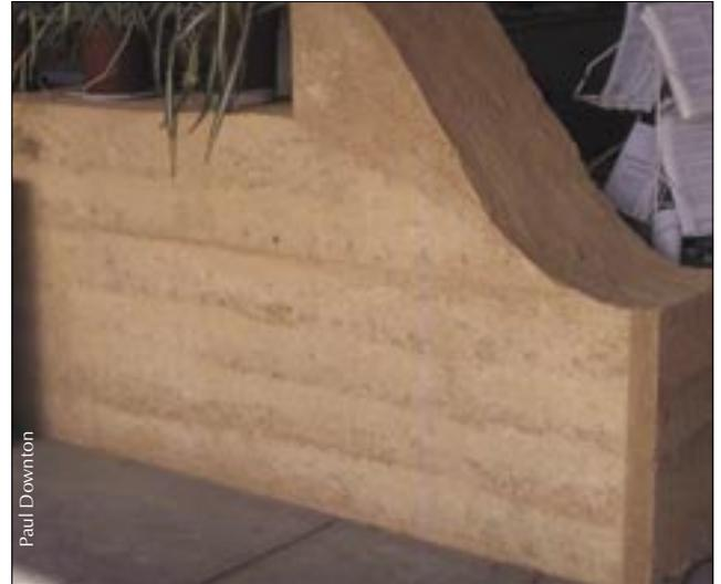
*In this sample wall the layers of ramming are visible as are the chamfered corners that are required to allow the walls to be easily released from the formwork. A part of the wall has been formed with vertical curves, made by carefully ramming along a drawn guideline on the interior of the formwork. Horizontal curves are also possible but require specialised, and therefore expensive, formwork.*
