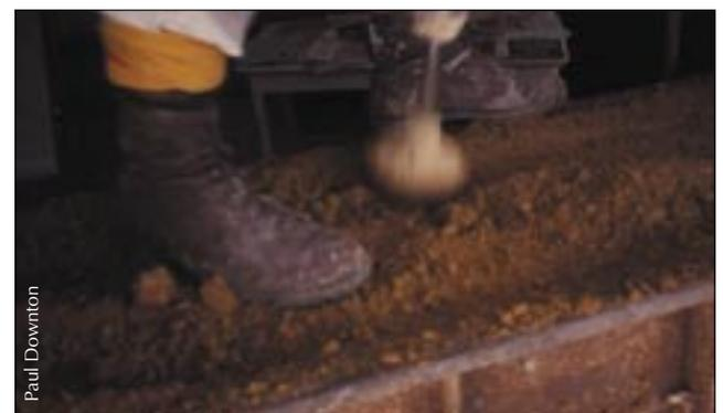
*Rammed Earth is made by ramming a mix of selected aggregates into removal formwork to create a monolithic, high mass wall. The modern process of making stabilised rammed earth is both labour intensive and highly mechanical, requiring the use of powered rams.*
