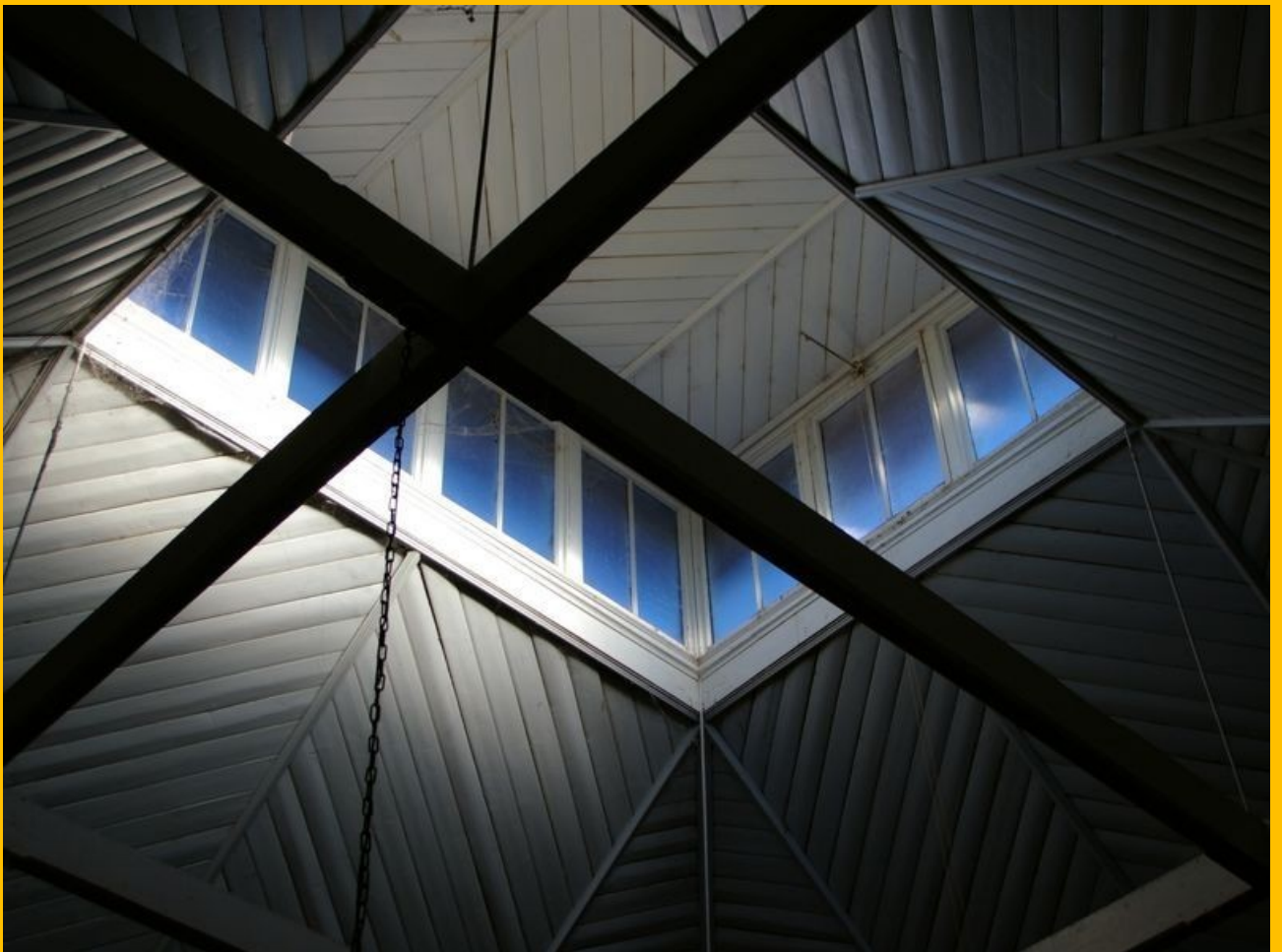
Ornate central skylight
