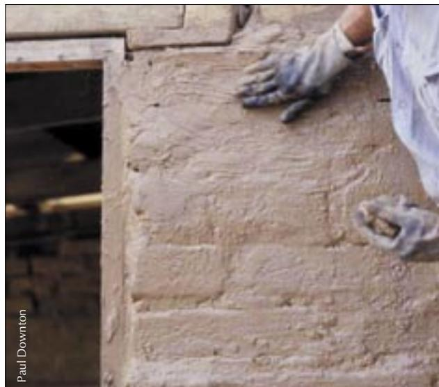
*After brushing to get a fairly even surface, the final finish is a mud slurry, typically finished by hand. This slurry may also be the final waterproofing coat (eg. A mud and cow dung mix) or it may have a further clear coat of proprietary waterproofing material. Linseed oil and turpentine can be used to provide a final finish.*
