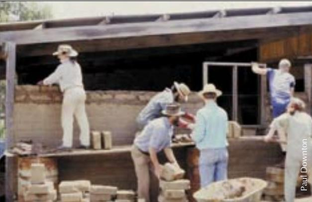
The **clay content** of adobe can range between 30 and 70 per cent and the overall earth content may also include silt, gravel and stones. There are a number of tests for suitability of the earth and the approval process may require an erosion test. Before excavating for on-site mud, consider the site layout to minimise carrying and transport and ensure there is space to keep any topsoil separate for use on the garden.
