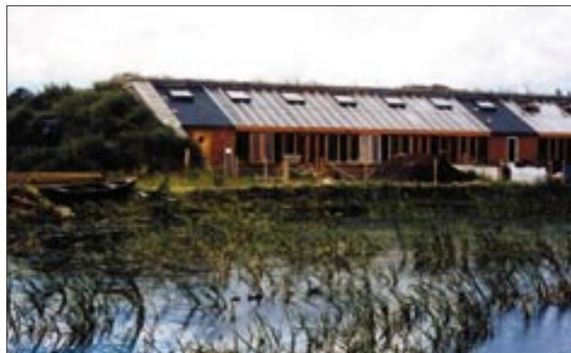
northern hemisphere). The earth that was excavated for the construction of the houses was put back on the roof.
