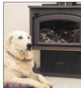
**An efficient wood heater** was installed for ambience and space heating – cost \$1500. Wood is a renewable energy source but the owners go to great lengths to ensure the wood they buy comes from a sustainable source. Wood is kept dry and the heater burns cleanly because they only turn it down after it has burnt hot for at least an hour. Tell tale creosote stains on the chimney appear when the heater is not burning efficiently. [See: [Heating & Cooling](#)]
