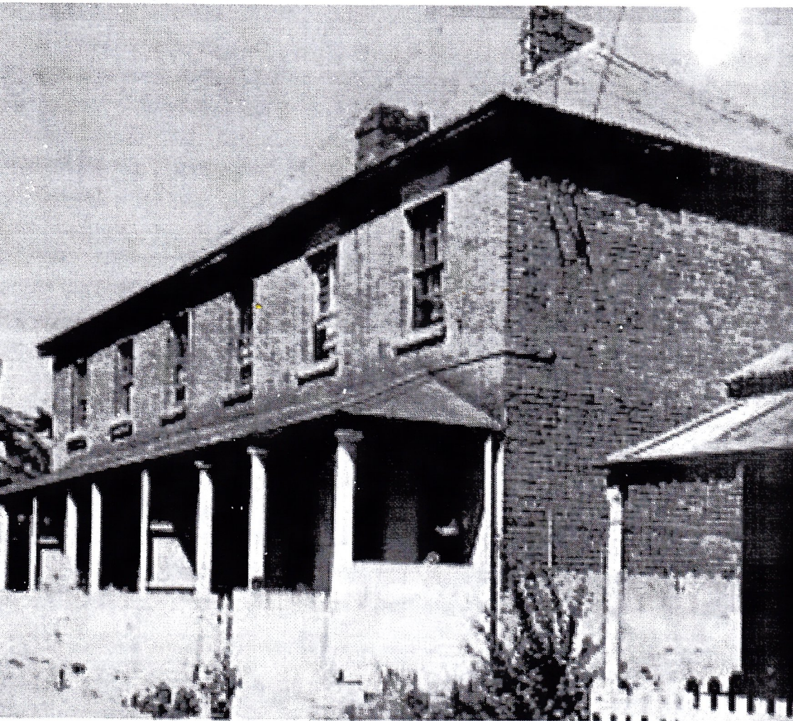
Terrace Houses Windsor 1830
