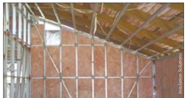
These bio-soluble batts are manufactured from around 30 percent recycled glass
