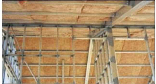
**External walls:** R1.5 pink wall batts™ with reflective foil laminate sarking as a vapour barrier. In hot climates the vapour barrier is usually placed on the outside of the insulation rather than the inside as this is where the condensation forms, particularly when internal spaces are air conditioned.
