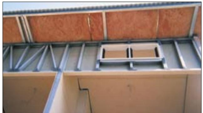
The eaves are also insulated in this climate to reduce radiation transfer through windows and walls.
