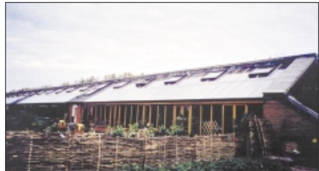
**The building envelope** is clay brick for exposed exterior walls and concrete internally. This maximises thermal mass and minimises maintenance. The south-facing conservatories use timber frames and glass, and the entrance porches have slate roofs. The planned building life is several hundred years. Passive Solar Heating, Lifecycle
