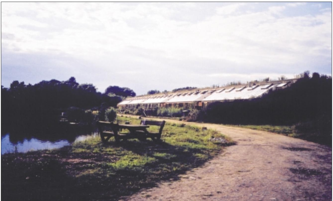
Production. Construction waste was minimised by the modular design. No spoil from the excavations left the site as it was all used to bury the houses. Now that the houses are occupied, the tenants have a communal composting system for organic waste of all types. [See: [Thermal Mass; Waste Minimisation](#)]
