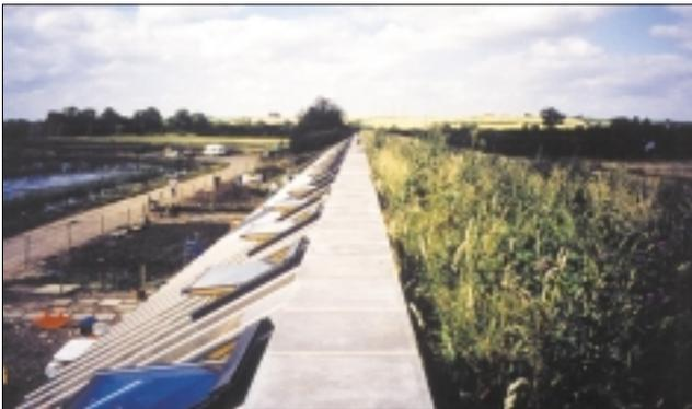
**Ventilation** for the houses is provided by opening windows in the external wall and glazed roof of the conservatory and opening windows and glazed doors between the house and the conservatory. In addition, each house has a mechanical ventilation heat recovery (mvhr) system that supplies fresh air to the living rooms and bedrooms and extracts from the kitchen and bathroom areas.
