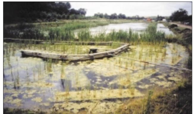
**The mats** are arranged with baffles in the water that form a spiral path for the waste water flowing through, and the waste water inlet is at the centre of the spiral. The pond is at one end of a large lake constructed for the project, and overflows into this lake.
