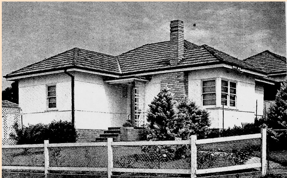
Austerity fibro house Note the small windows as glass was still scarce
