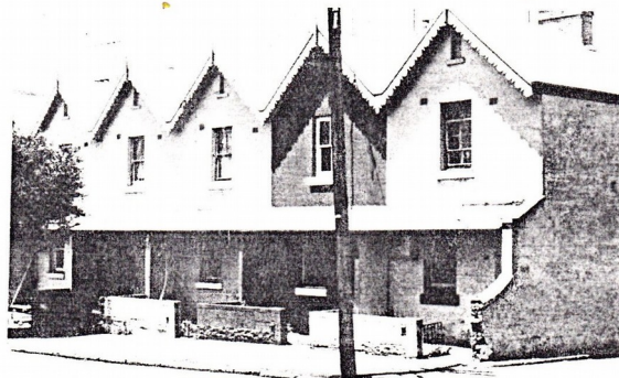
Louisa Terrace, 124-134 Mitchell Street (1875). Post-Regency, but with features of the Picturesque style: carved bargeboards and 'dove-cote' recesses in the gables. Park Terrace, across the street at 101-111 Mitchell Street, is virtually identical.
