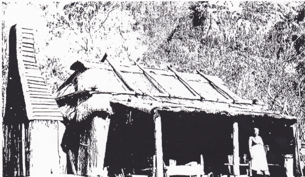
Early settlers house - early 1800s The timber structure on the bark roof is to stop the bark curling up
