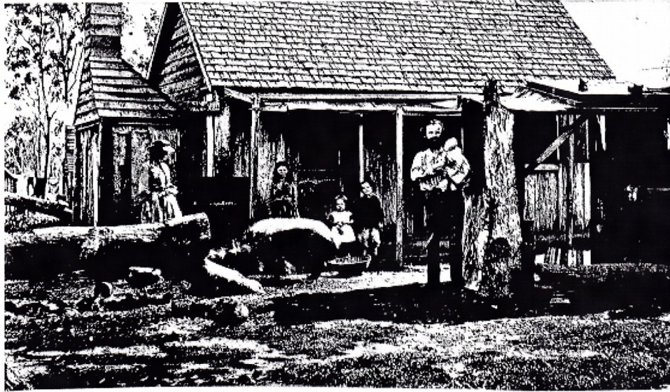
Settlers house - early 1800s Wooden shingles have replaced bark roof
