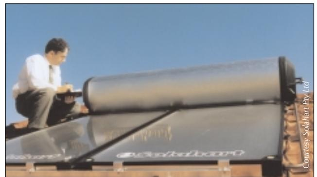
**Solar hot water systems** are storage systems and, depending on your climate can provide up to 90 percent of your hot water for free using the sun's energy. Solar systems may be less appropriate in smaller households, in cooler parts of the country, or where access to sunlight is restricted. [See: Solar Hot Water]
