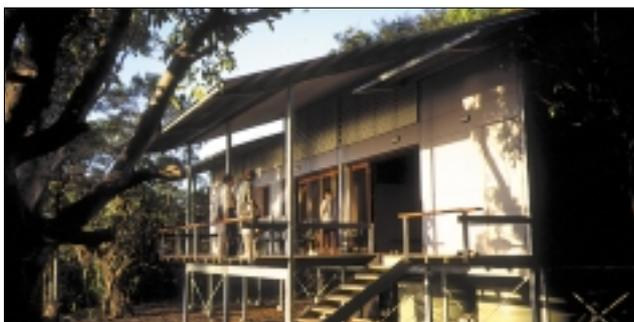
**Roofing** and ceilings are in corrugated steel sheet on steel purlins.
