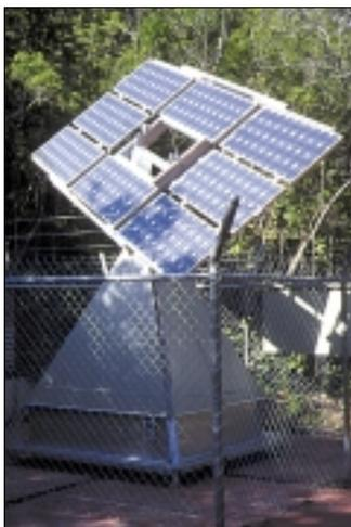
A Remote Area Power Supply (RAPS) system is installed. The system used is a commercially available system (Pyramid Power). This includes a solar tracking array of Photo Voltaic (PV) cells, an inverter, a battery bank and a backup generator. The batteries and control system are mounted in a pyramid shaped storage box underneath the panels. The backup generator is rarely required.
