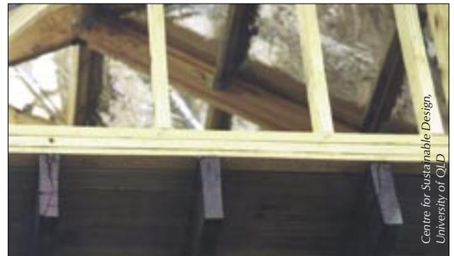
**De-nailed**, stress graded, recycled structural hardwood and decking timber was used to reduce embodied energy. Timber doors and windows from sustainable forest plantation hoop pine were installed throughout the home.
