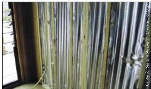
**The aluminium foil insulation** shown above with a 25mm reflective air gap each side stops 97 percent of radiant heat. It is economical, efficient, non-irritant, non-allergenic and recyclable. An under roof insulation blanket provides condensation insulation to the steel clad roof and walls.
