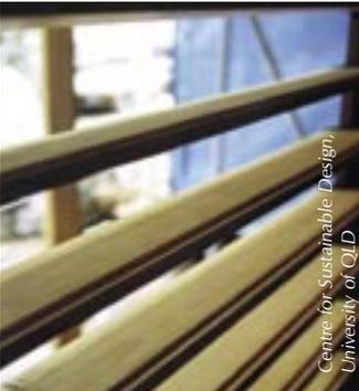
**Maximum north facing** timber windows, timber bi-folds, french doors and louvers with a blue azulite tint glazing are used. The high performance glass absorbs a significant amount of the sun's near infra-red heat energy and reduces the transfer of heat into the home. [See: [Glazing Overview](#)]
