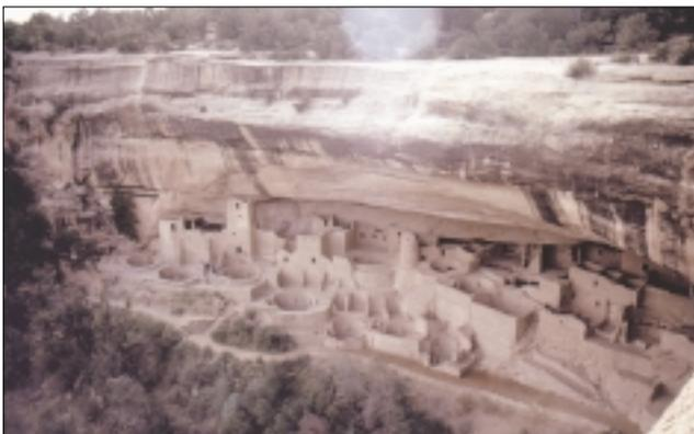
**Ancient cliff dwellings of American Indians** in Mesa Verde exploit the cliff overhang for full passive solar control to not just the walls and windows, but the whole village. Natural updrafts provide excellent ventilation. Buildings are of adobe and rock - high in thermal mass, low in embodied energy.
