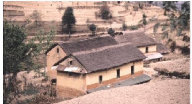
**Passive solar orientation and shading** maximises solar gain. East and West glazing is omitted. Walls of rock collected from farm terraces are high in thermal mass and blend with the landscape (they are annually rendered with mud in colours of the landscape). This guarantees longevity and prevents heat loss by caulking cracks and crevices. Early Australian settlers used similar building methods. [\[See: Passive Solar Heating\]](#)
