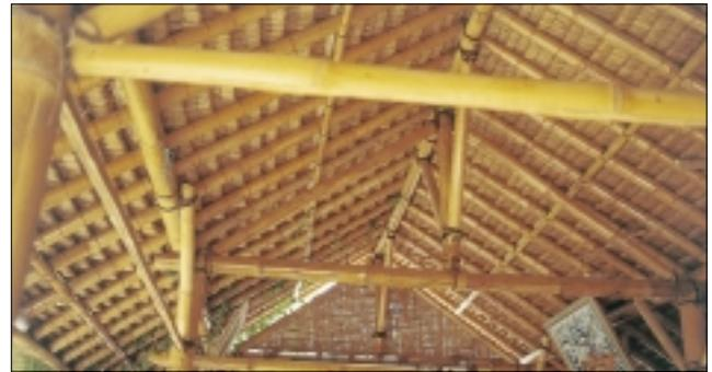
**Indonesian vernacular buildings** use thatch as high level insulation to deal with heat gain in a tropical climate. Open gables allow cross ventilation of the hottest air that would otherwise accumulate in the roof space. Generous eave overhangs shade the building, further reducing heat gain. These principles are employed in the traditional "Queenslander" which is also an excellent example of climate responsive architecture.
