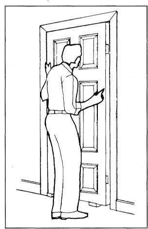
TRIM DOOR: Remove door from frame and with hand plane, power planer, hand or power saws, as available, trim back to clearance lines marked in Step 3. If stock size doors are too narrow for the opening, then margin strips can be glued and nailed to the edges of the door to make up the required width. Naturally, matching timber is desirable where appropriate and the piece should be planed and sanded to give an exact fit.
