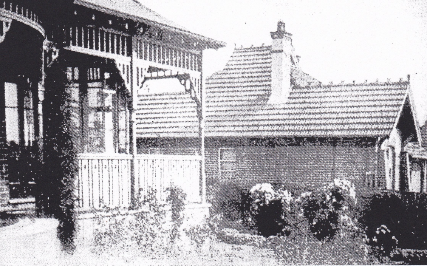
Federation houses in Haberfield. Shows the attractive verandah fretwork typical of Federation verandahs
