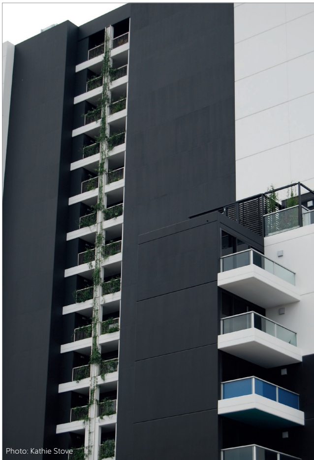
Greenery can be part of a high-rise apartment block.
