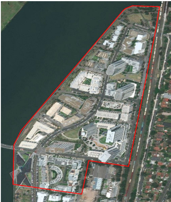
Figure 26: Aerial photo of case-study precinct, showing boundaries
