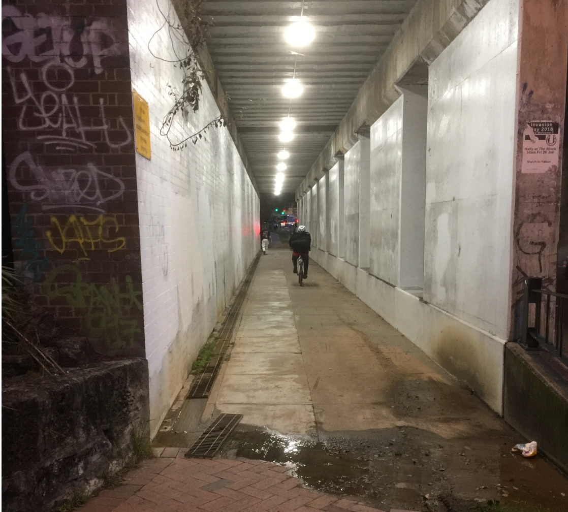
Figure 37: Pedestrian underpass to Strathfield commercial centre
