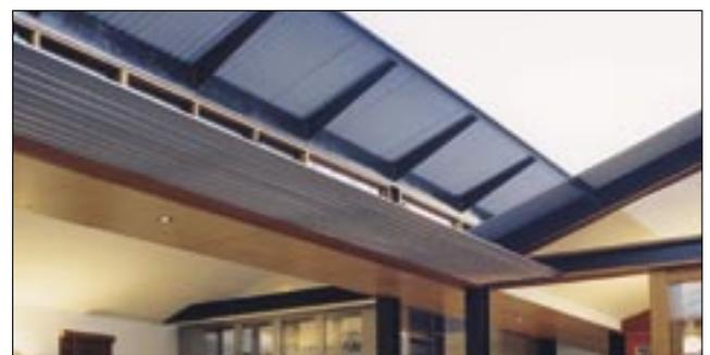
**Pre formed horizontal metal louvres** over the doors are set to an angle that allows deep winter sun penetration whilst excluding summer sun. More sun is gradually allowed into the house as winter approaches, providing an interesting pattern across the floor and walls as a reminder of the time of year.
