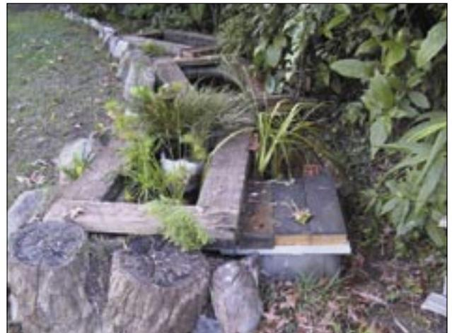
The waste water is fed up through this matrix, overflowing at one end into the bottom of the next tank, where the same process is repeated, and again into the third tank.
