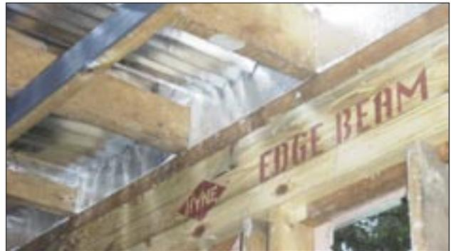
**Engineered timber** allows these longer spans to be handled with minimal member depth. A laminated 200 x 45 mm timber beam called a *Hyne Edgebeam LGL* was used in this instance.
