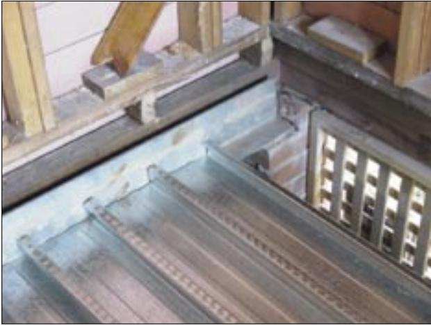
**This type of slab** uses the existing piers and footings, and requires no filling or excavation. The concrete is poured over prefabricated steel decking. The slab was installed lower than the original floor to gain extra ceiling height.
