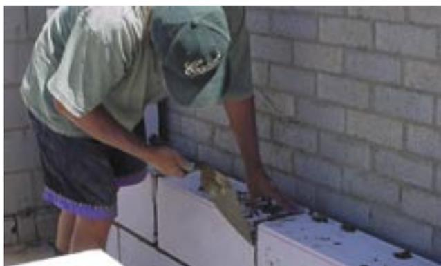
**AAC is laid in a similar manner to conventional masonry. This illustration shows 'thick-bed' mortar (about 10mm) being used, but thin-bed AAC joints are only 2mm or so and the end result behaves more as a monolithic wall.**
