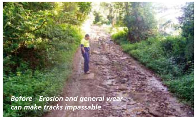
*Before - Erosion and general wear can make tracks impassable*
