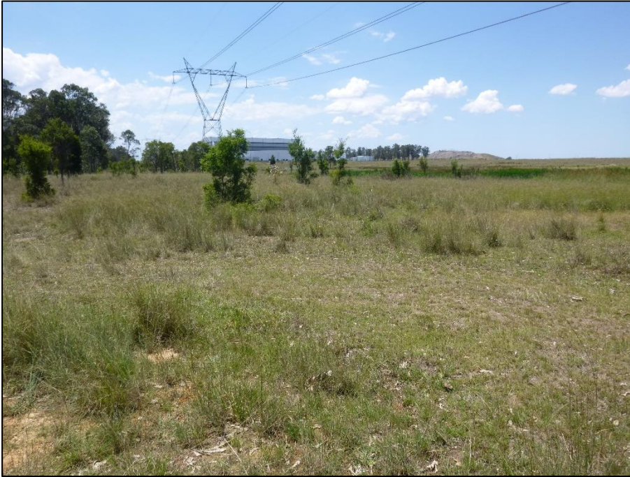
View north along the 330kV Electricity Transmission Line through the Study Area
